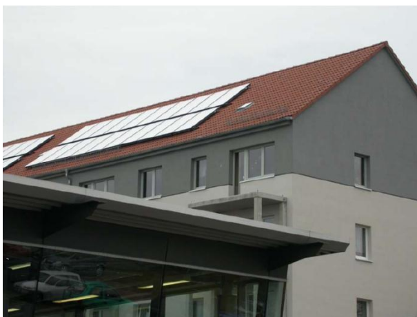
Figure 1: Grünstraße solar heating system (source: Parabel Energiesysteme GmbH)
