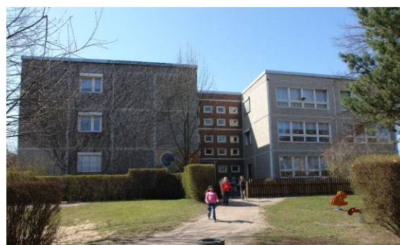
Children’s day care centre “Burg” in Luckenwalde
