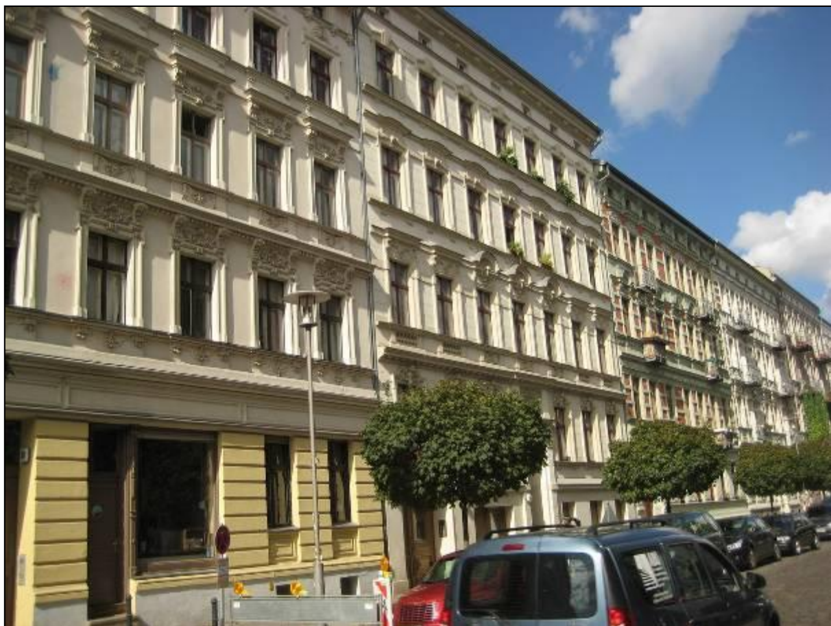
Fig. 29: Refurbished façades in Pfarrstraße (2010)
