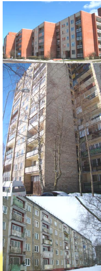
Pic.6, typical multi-apartment buildings in Jugla
