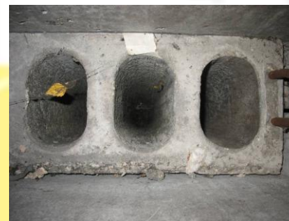
Pic.14, clean ventilation shafts (multi-apartment building of series No.464). [9]
