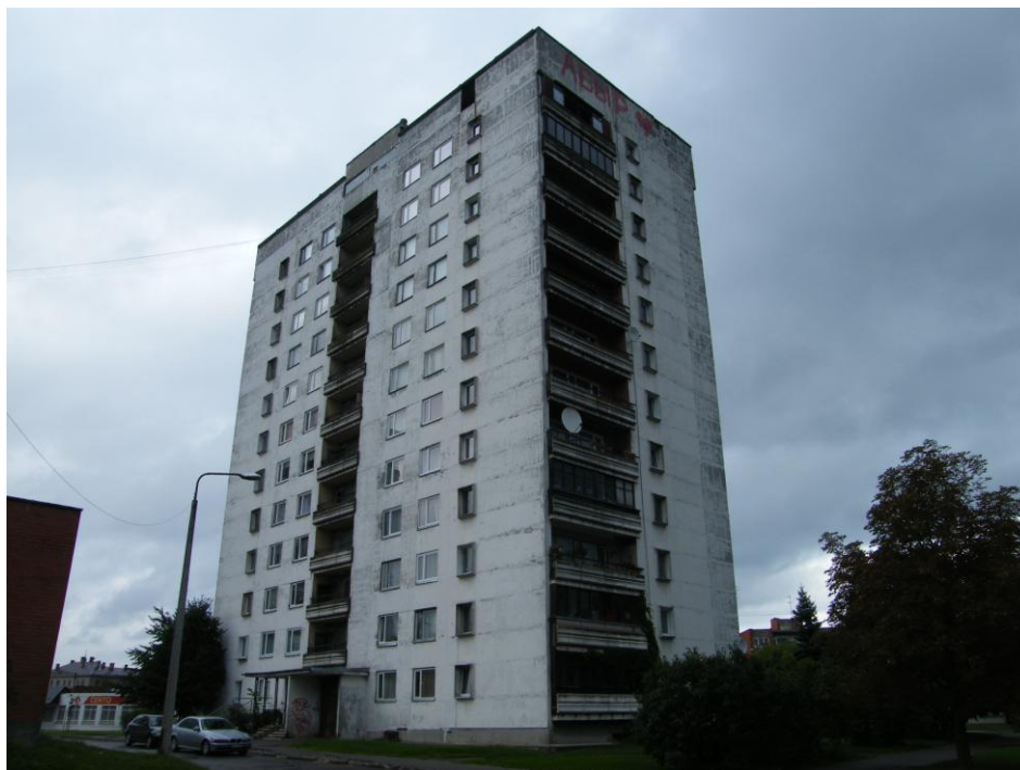
104th Series - 12-story residential building at Pasta Street 38
