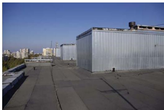
Fig. 4. Roof of Apartment Building No. 11 in Sevastopolio Street
