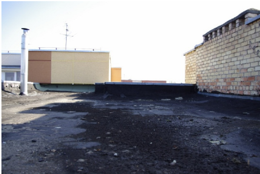
Fig. 4. Roof of Apartment Building No. 156 in Vytauto Street
