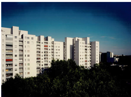
The quarter Märkisches Viertel will be refurbished to Germany's largest low energy quarter Photo: GESOBAU
