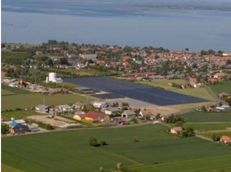
View of the Marstal solar collector area in Denmark Photo: Leo Holm, Marstal Fjernvarme.
